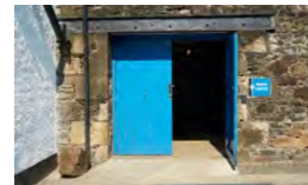
The mash house entrance
